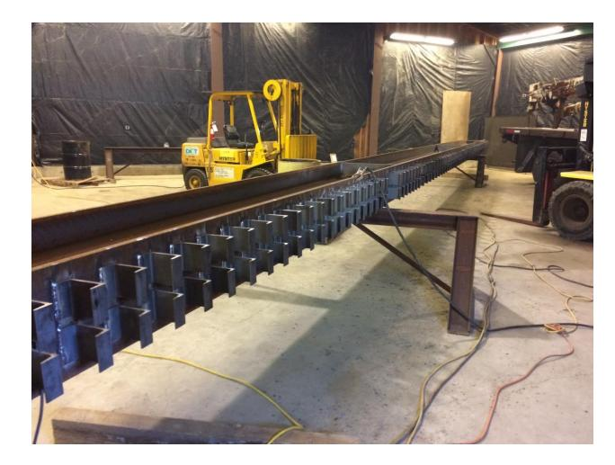
The use of heat and/or jacking has been used to for decades to repair distortions caused by welding, install camber in bridge girders, and induce horizontal curves in bridge girders.
