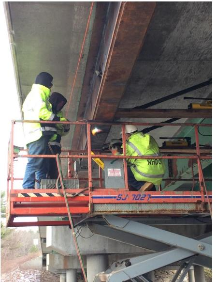
Heat-straightening is a repair technique conducted in the field for steel that has been damaged, and portions have exceeded the yield stress
